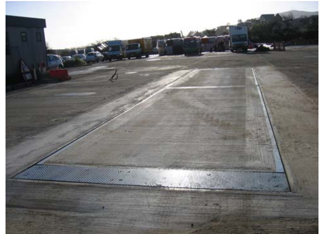
Concrete finish up to the channel surround leaves a tidy installation
