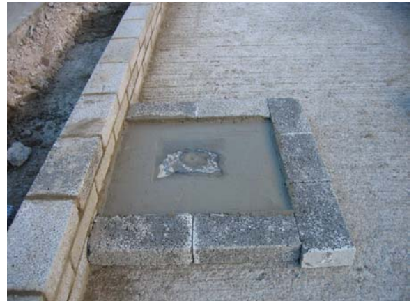
Six plates with 300mm x 400mm steel plate cast into foundations
