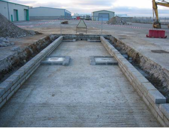
Foundations prepared by builder
