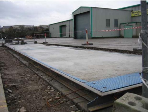
Deck in place with channel surround
